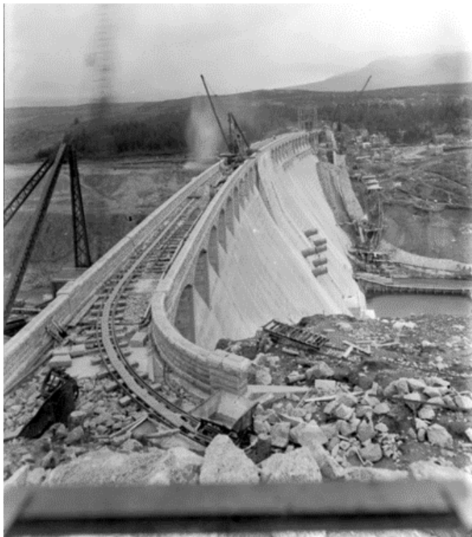
The construction of Laggan Dam
